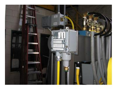
Adjustable differential - Difference between the trip and reset values
